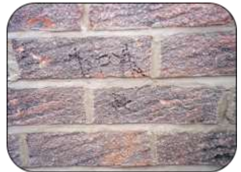
Brick stairwell sealed with 2 coats of 556 Clear cladding
