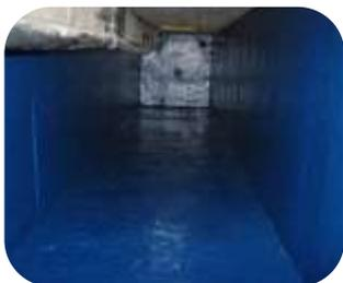
**Resichem 573 Fastfill Screed** is a single component fast curing engineering grade, polymer modified, reactive cementitious coating with high adhesive properties. It is used in permanent immersion or negative pressure waterproofing. It incorporates the most advanced micro-silica, polymer and fibre technology, curing to give a dense matrix which is impermeable to water under 10 bar hydrostatic head. Supplied as a single component system, ready for on-site mixing and use.
