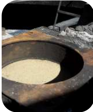
Process equipment foundation at a steel plant rebuilt using 576 Quartz Screed
