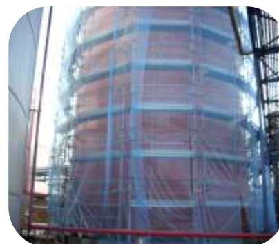
Petrol storage tank at European refinery hydroblasted and coated with 2 x coats of Resichem 555 Resinox
