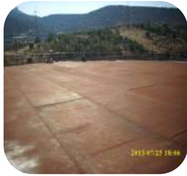
Crude oil storage tank roof was cleaned with high pressure water at 1000psi. Resichem 555 Resinox was applied in 2 coats at 500 microns wet film thickness per coat.
