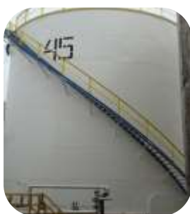
Petrol storage tank at European refinery hydroblasted and coated with 2 x coats of Resichem 555 Resinox
